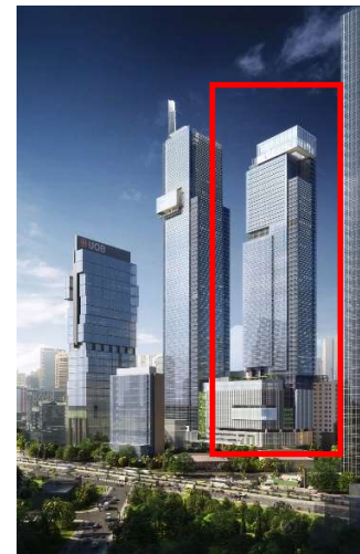
Luminary Tower (Right)
