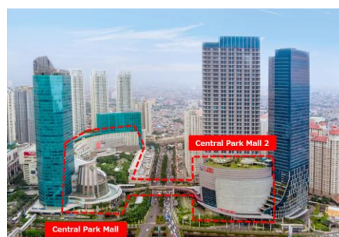
Exterior view of the building
